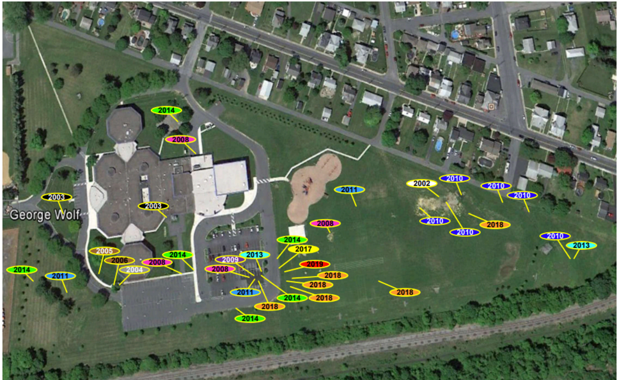
Figure 24 – Sinkholes at George Wolf Elementary School
